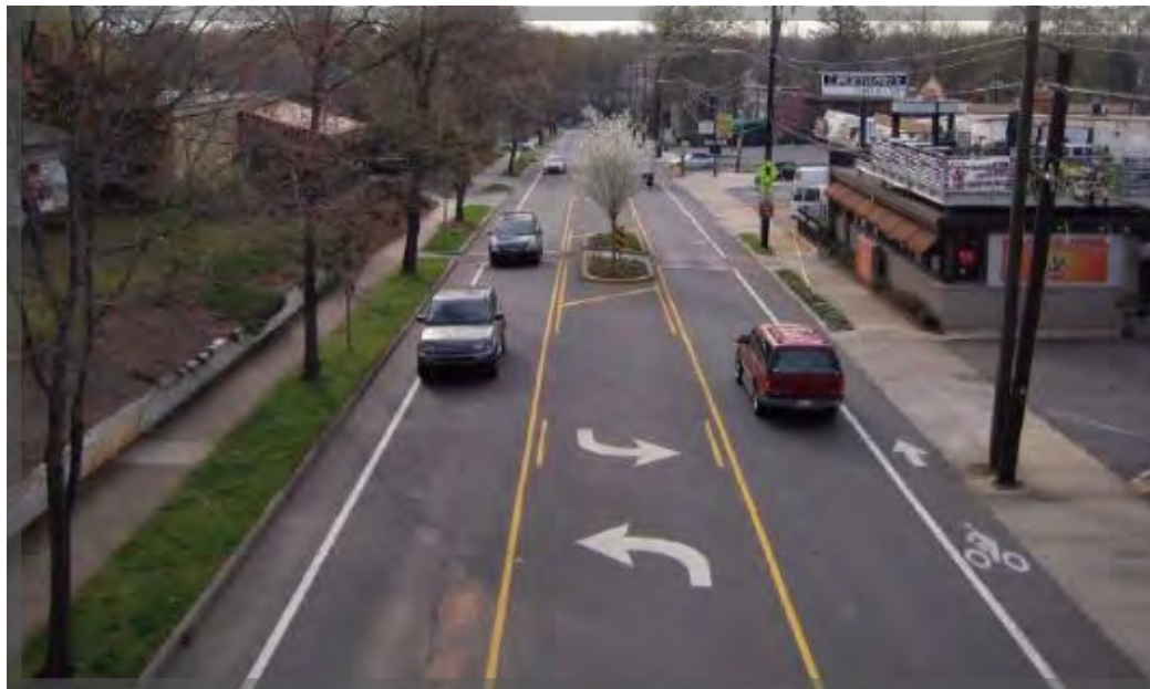
Example of a Middle Turn Lane in the Midwest
