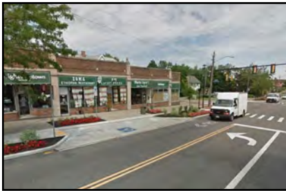
Cedar Road; turn lanes, parking & plantings
