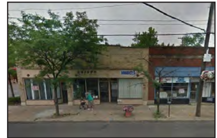
Noble Road; typical condition
